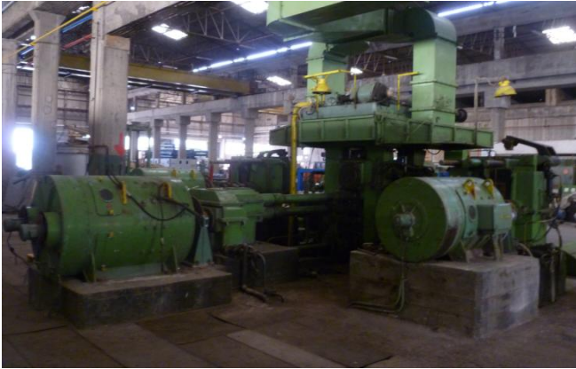
View of the industrial installation
