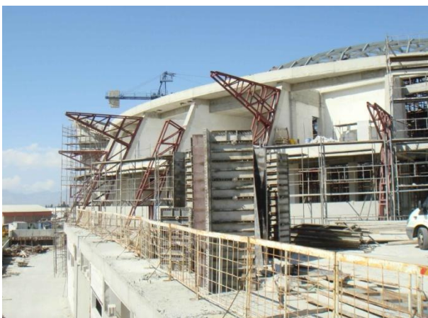
Scaffolds covering the site
